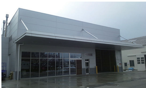
Biomass power generation facility
