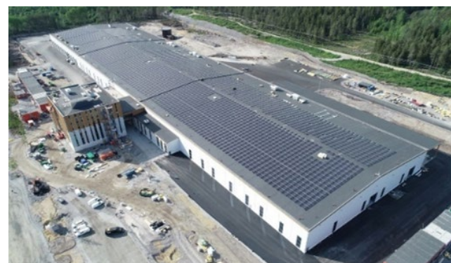
Solar panels of the new plant
