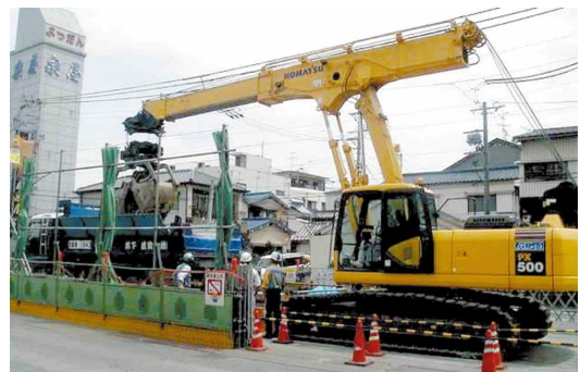
Photo 8 PX500 in action at a subway system construction work site
