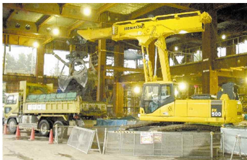
Photo 7 PX500 in action at a construction underground work site
