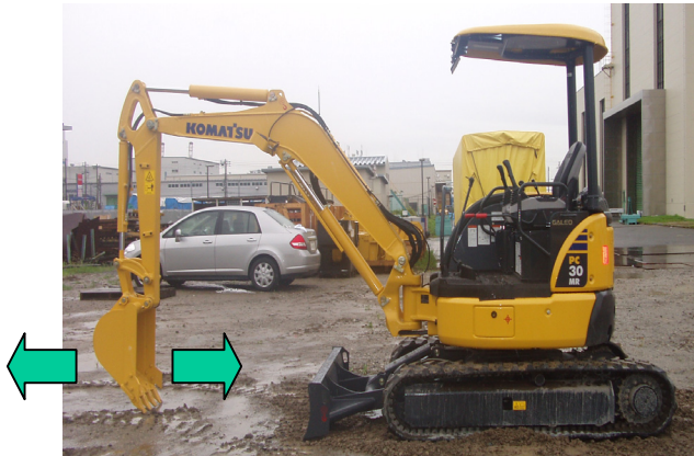
Photo 3 Rough plowing (finishing) work
