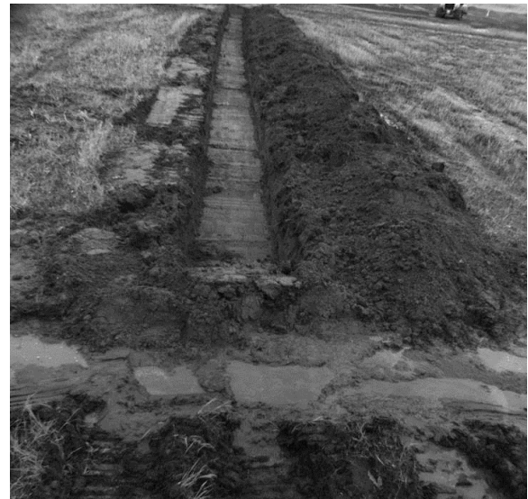
Fig. 9 Photograph of jobsite taken by stereo camera
