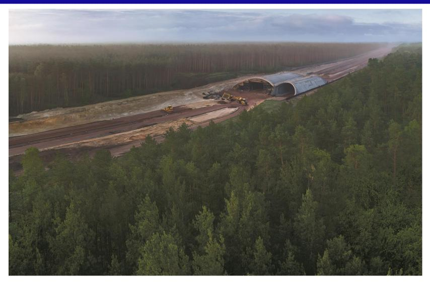
German highway construction site with smart construction On building an animal bridge connecting the forests to protect the ecosystem
